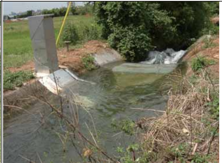
Precision level transducer TW-252S used for flow monitoring on a long-throated flume.
